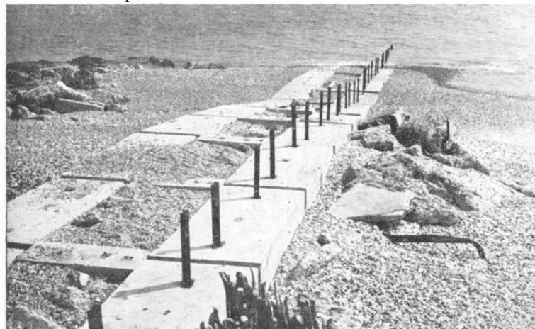
Fig. 11 Selsey Bill. Articulated concrete groyne
